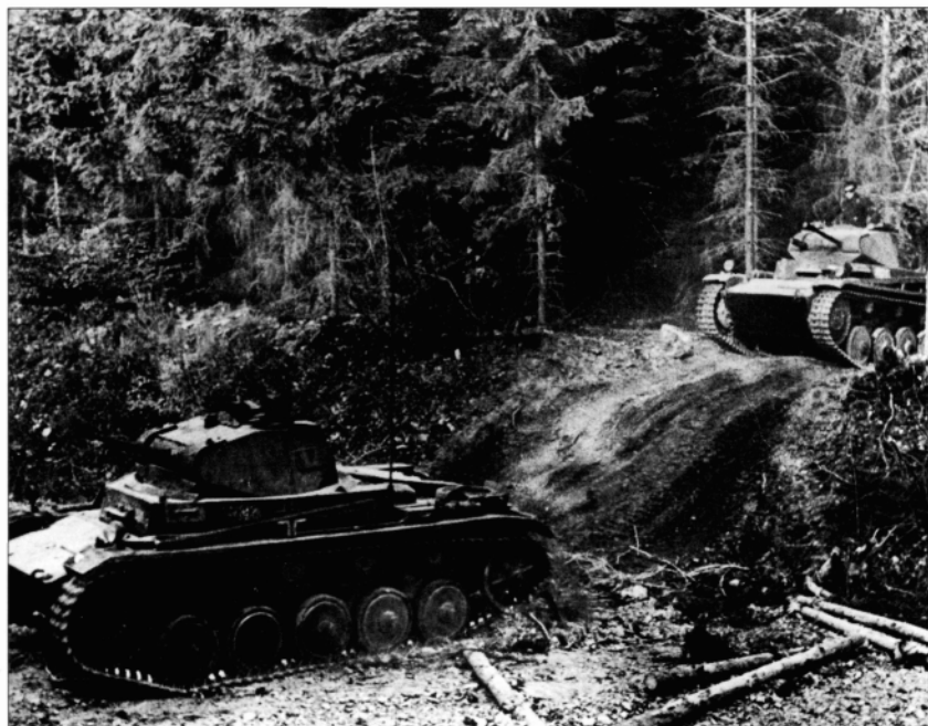
Two PzKpfw II Ausf c training in woodland. The Ausf c was the first variant of this tank, produced from March 1937; it featured a new suspension system, with five independent large road wheels and new tracks.
